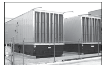
8,000 Gallon Subbase Tanks
