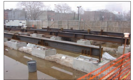
A “cushion” helps meet seismic requirements. Custom steel spring isolators separate the building from the subway structure, attenuating vibration and sound from moving trains. Also, the steel sits on Teflon so the building can slide over the subway structure in the event of shock loading.
