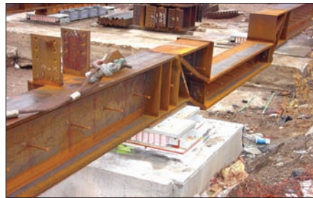
A “cushion” helps meet seismic requirements. Custom steel spring isolators separate the building from the subway structure, attenuating vibration and sound from moving trains. Also, the steel sits on Teflon so the building can slide over the subway structure in the event of shock loading.
